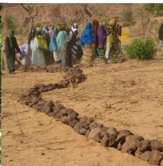
Construction of stone bunds, Niger © PASP, GIZ
