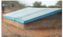
Underground storage tank
